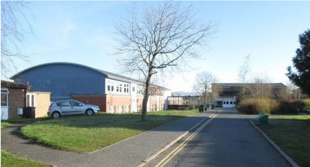
Figure 3: Ysgol Calon Cymru Llandrindod Campus
